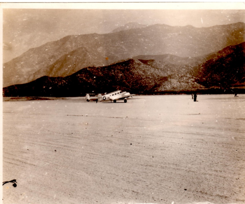
BANNING, CALIFORNIA 31 AUG. 1943 THE BANNING LANDING STRIP WAS THE BATTALION'S FIRST CONSTRUCTION TRAINING. ABOVE, THE PARKING APRON.
