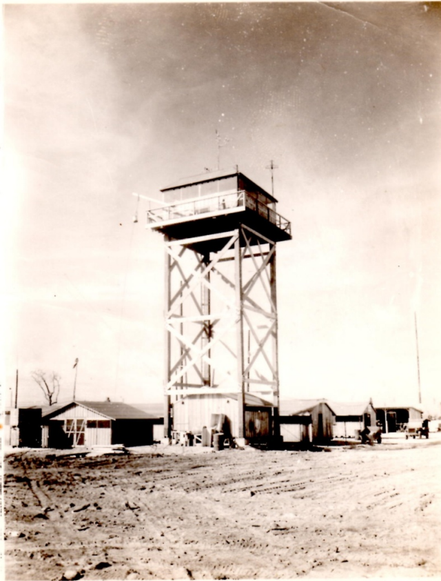
KWAJALEIN 26 MARCH 1944 THE PERMANENT CONTROL TOWER STANDS COMPLETE AND IN OPERATION AFTER 25-FOOT MOVE INTACT.
