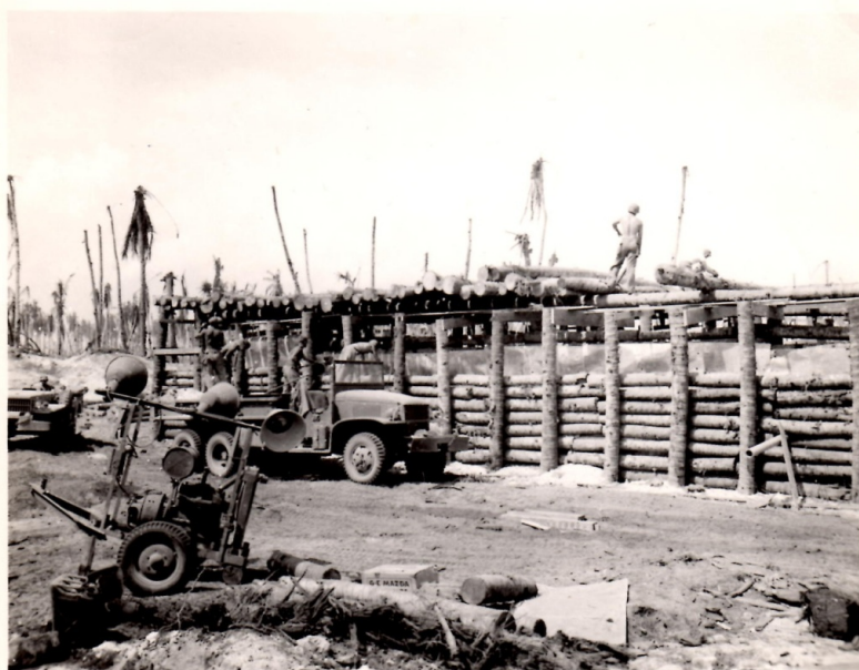
KWAJALEIN 17 FEBRUARY 1944 BUILT OF PALM LOGS AND SAND FILLED WALLS, THE FIGHTER CONTROL BUILDING NEARS COMPLETION.
