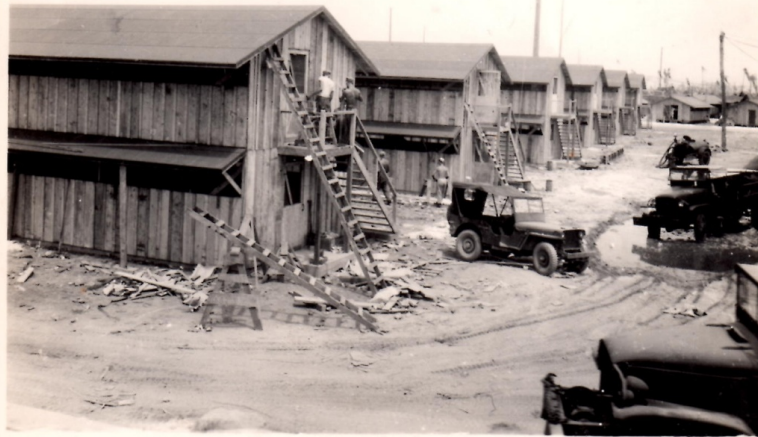
KWAJALEIN 15 MAY 1944 LAST STAGE IN ASSEMBLY - LINE CONSTRUCTION IN THE 11TH BOMB GROUP HOUSING AREA.
