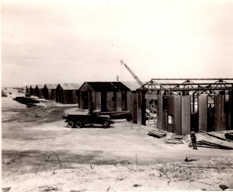
KWAJALEIN 19 MAY 1944 SEVEN OF THE 14 STEEL WAREHOUSES ERECTED FOR THE HAWAIIAN AIR DEPOT BRANCH.
